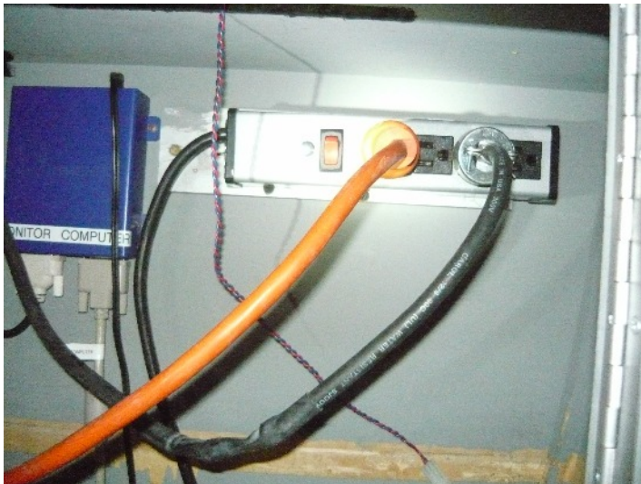
And of course the obligatory Power strip to power everything up
